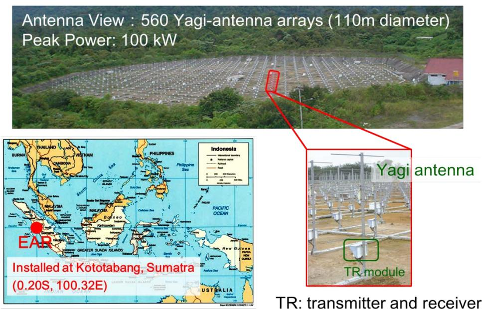
**Figure 1:** Overview of EAR (top) with configuration of each Yagi antenna (bottom right) and location of the EAR site (bottom left).
