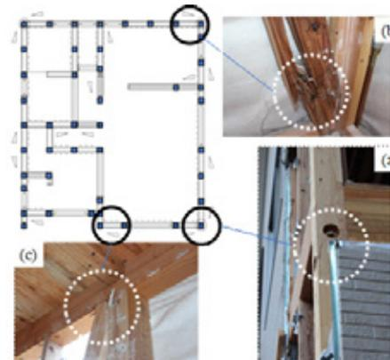
Figure 2. Observed damage to the test building with minimum requirement.
