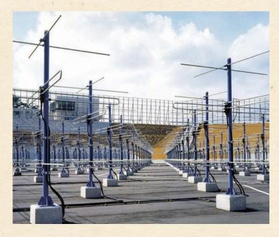
The MU radar uses VHF radio waves with a frequency of 46.5 MHz (1 MW peak output power). The antenna area consists of 475 Yagi antennas arranged in a 103 m diameter circular array. Fast beam steering and flexibility for various observational configurations characterize the instrument.
