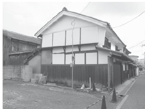
Fig.4 Outside view before renovation
