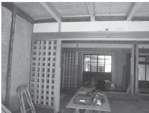
Fig.3 Inside view of the house under construction.
