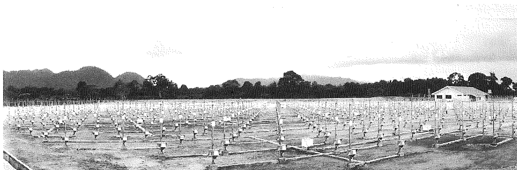
Fig. 1. Picture of EAR installed at Koto Tabang, West Sumatra, Indonesia
