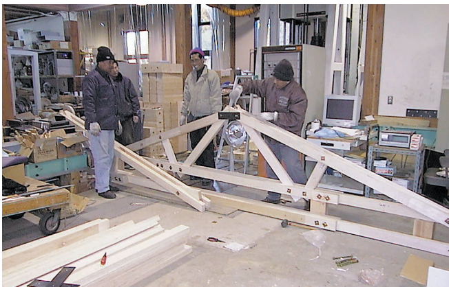
Assembly of LVL truss members
