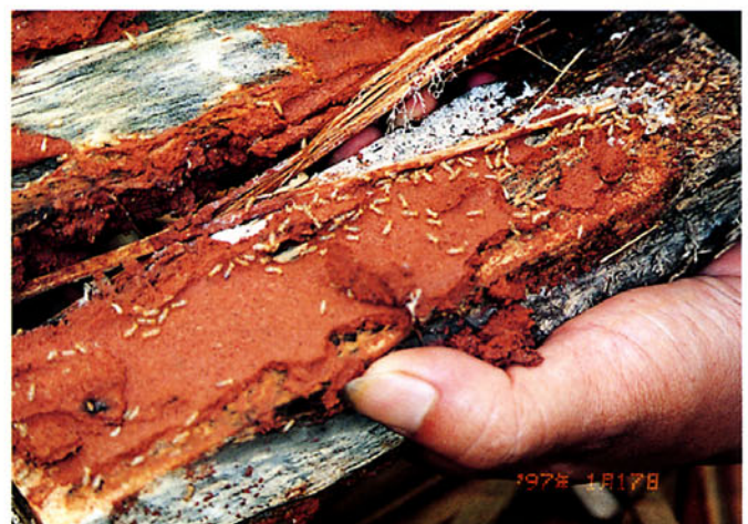
Fungus-growing termites attacking timbers in a field test site at Serpong
