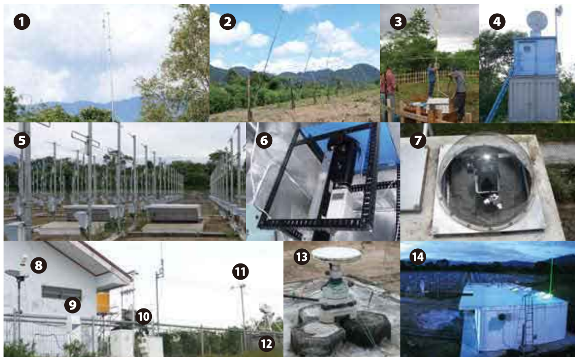
Figure 3: Equipment installed at the Equatorial Atmosphere Observatory. ( ① FM-CW ionosonde, ② VHF radar, ③ Meteor radar, ④ X-band meteorological radar, ⑤ RASS speakers, ⑥ All-sky imager, ⑦ Fabry-Perot interferometer, ⑧ Micro-rain radar, ⑨ Ceilometer, ⑩ Disdrometer, ⑪ Optical rain gauge, ⑫ Radiometer, ⑬ GPS receiver, ⑭ Lidar )
