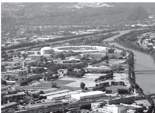
図4 The European Synchrotron Radiation Facility.
