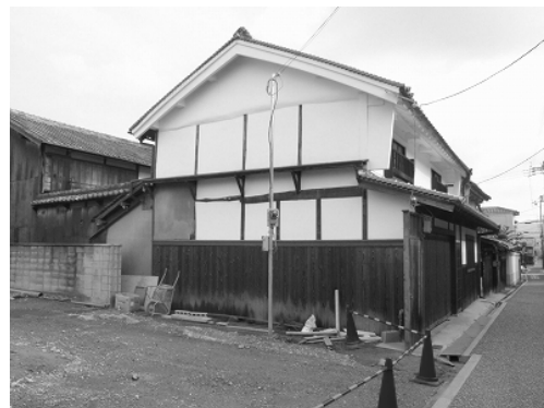
Fig.4 Outside view before renovation
