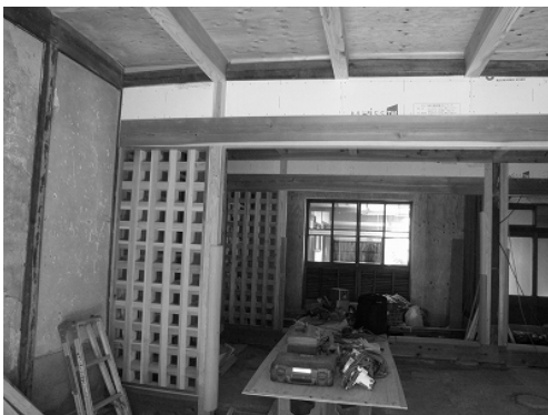
Fig.3 Inside view of the house under construction.
